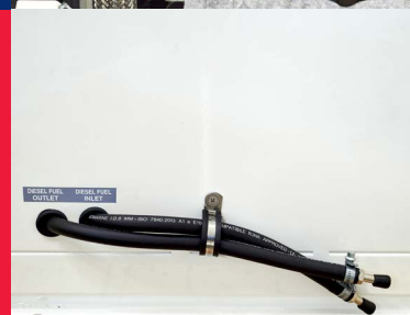
Fuel inlet and outlet
